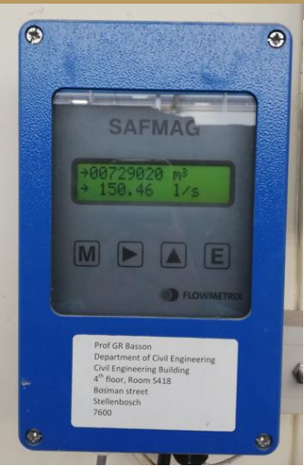
Flowmetrix SAFMAG electromagnetic flowmeter used to measure flow (accuracy of ±0.5%)
